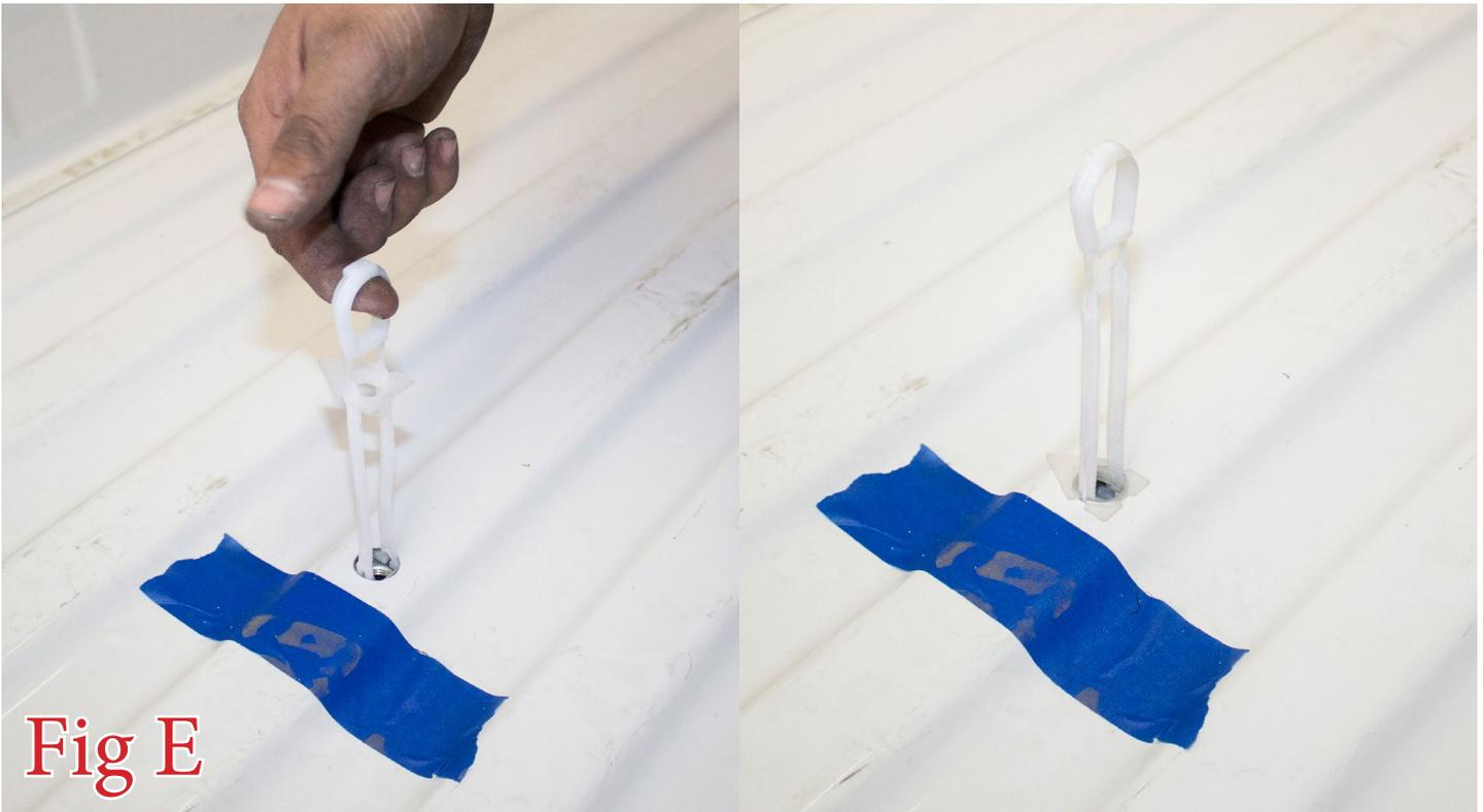
6. With the snaptoggle in place, break the lines off so it looks like (Fig F).
